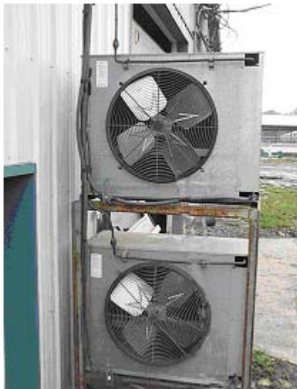
Figure 2-4. Remote air-cooled condenser
