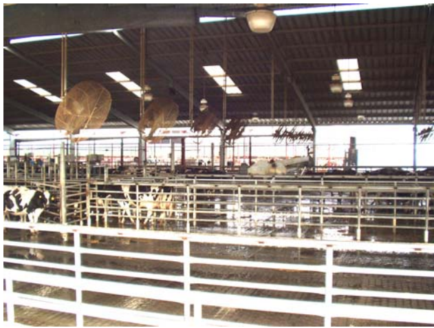
Figure 3-3. Lighting in parlor stalls, return lane lighting, and holding area lighting
