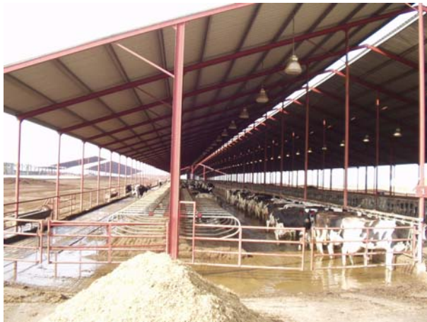
Figure 3-7. Freestall resting barn with supplemental long day lighting
