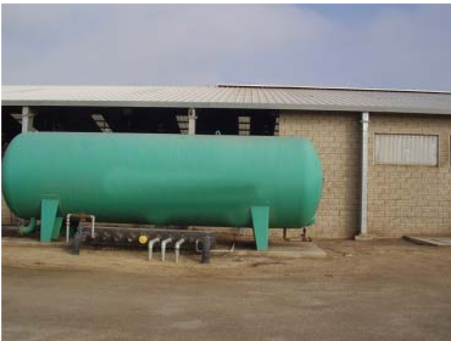
Figure 6-7. Pressure tank on California dairy
